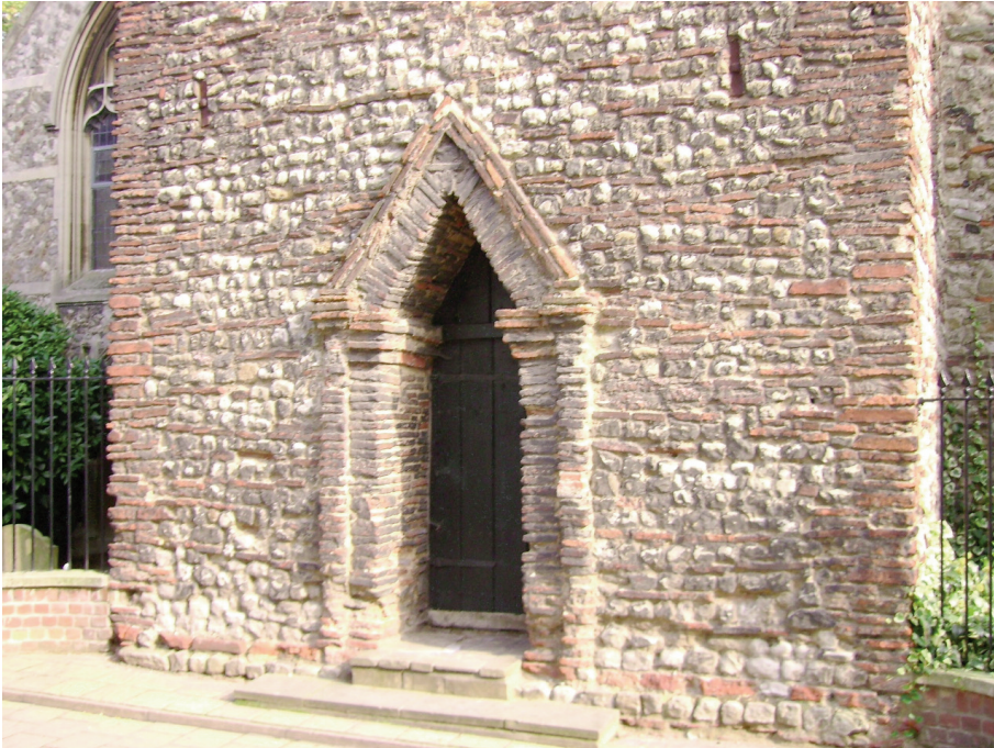
Fig. 1. 11 th -century doorway of Holy Trinity Church, Colchester, built with recycled Roman brick (photo Christian Etheridge, licensed under Creative Commons).
