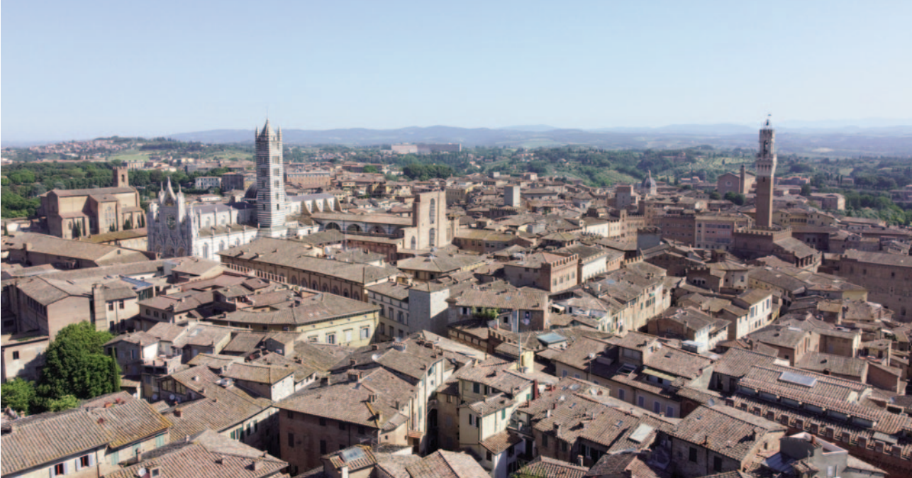
Fig. 1. Drone photograph of the town centre of Siena (Image: Gianluca Fenili).
